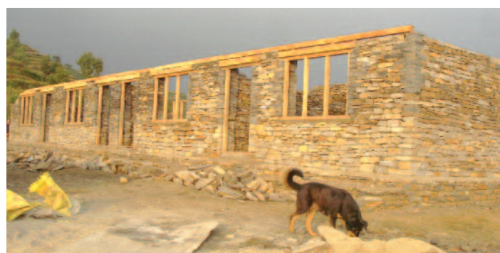
Ever improving 'Bradley Wood' building work in progress
